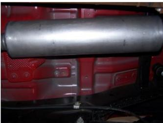
4. Install muffler #B onto headpipe 1½"-2" with the louvers facing towards the converter. Use a jack stand to support the muffler. Use clamp #E to secure the muffler to the headpipe. DO NOT TIGHTEN. Muffler inlet is looking into the louvers. Outlet of muffler will be at approximately 12 o'clock.
