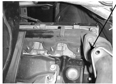
#6. FACTORY FLANGE CONNECTION. DISCONNECTING POINT.
